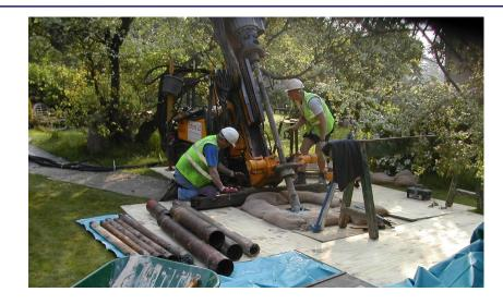
Site Investigation work comprising rotary open drill holes and rotary cased drill holes together with in-situ testing and down-hole geophysical surveys to determine the nature and extent of former mine workings within the Oolitic Limestone covering in excess of 50ha, at Combe Down.
